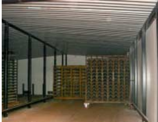
Fig. 6 Internal view showing the product and inclined roof to prevent any condensation drop out.
