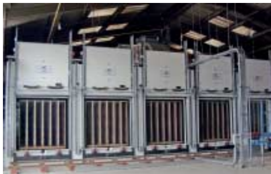
Fig. 1 Entry end showing 5 lanes forming the complete concrete curing system.
