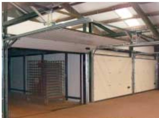
Fig. 5 External view of two batch loaded curing chambers for specials.
