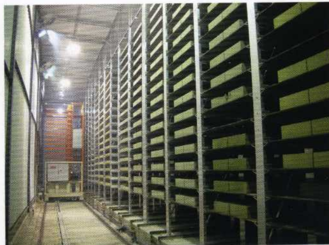
After collecting the pallets on the wet side, they are put into the curing racks by the finger car
